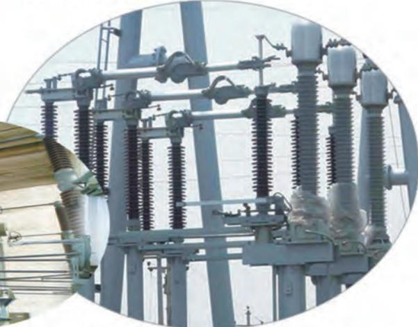
Open-type assembled switch series
